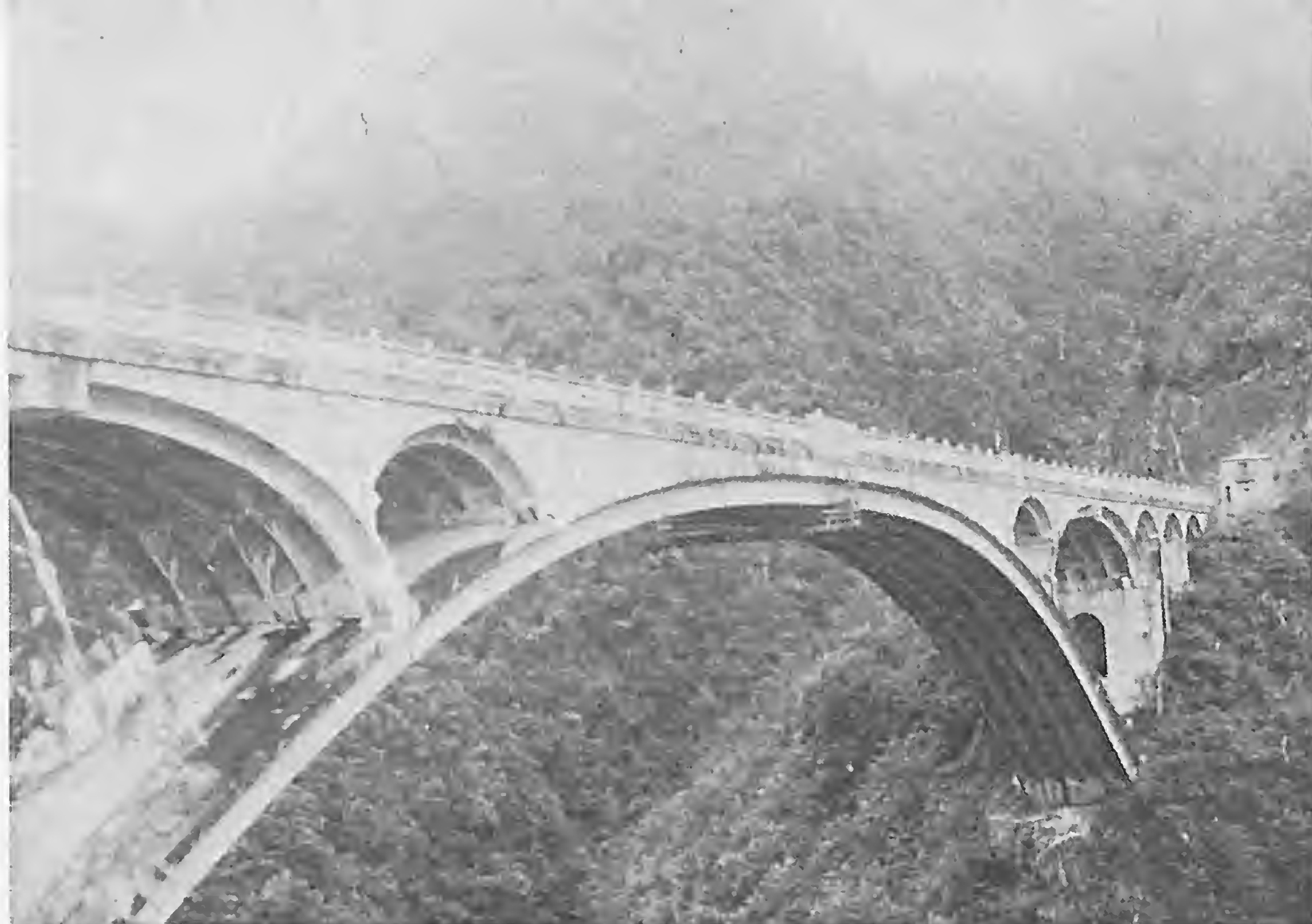
Open-spandrel bridge over a mountain valley.
